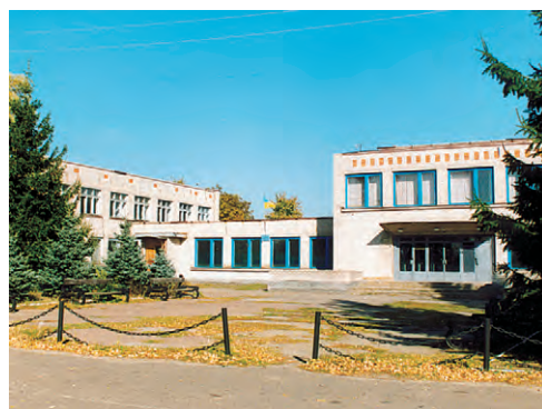
v. Rozumivka. The administrative building
